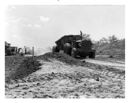
Detail of a bottom dump truck owned by the Grandview Company of Mount Vernon, NY. A bulldozer and workmen are also in view. The image is a construction progress photograph taken by the Dept. of Public Works, Bureau of Highways (related photograph file number 4966).
