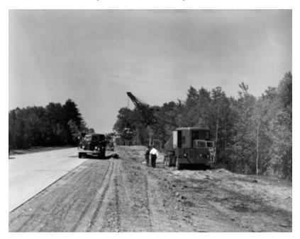
A crane and shovel operating at a point on Troy-Schenectady Road. The road is partially paved and wooded on both sides; a dump truck, car, and workmen are also in view. The image is a construction progress photograph taken by the Dept. of Public Works, Bureau of Highways, (related photograph file number 4967).
