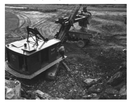
Detail of a Bucyrus-Erie cable shovel, owned by Lane Construction Corp., Meriden, Conn., loading rock in to a dump truck. Workmen are also in view. The image is a construction progress photograph taken by the Dept. of Public Works, Bureau of Highways (related photograph file number 5031).
