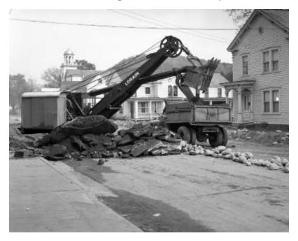
Lorain cable shovel emptying dirt into a dump truck on Main Street in Warrensburg. Road work is near First United Methodist Church. Houses line the street and Adirondack mountains are in the background. The image is a construction progress photograph taken by the Dept. of Public Works (related photograph file number 5168).
