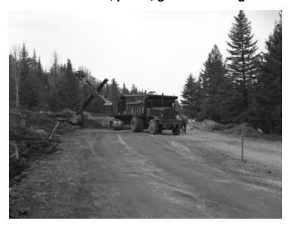
Bucyrus Erie cable shovel, dump truck, and workmen at a work site in a wooded area of Ballston Lake. The image is a construction progress photograph taken by the Dept. of Public Works, Bureau of Bridge and Grade Crossings (related photograph file number 5274).
