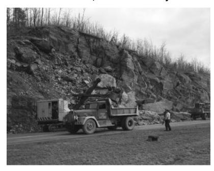
Cable shovel loading debris from a rock slide into a dump truck on a portion of the Catskill Thruway bordered by a steep rocky incline. Two workmen look on nearby. The image is a construction progress photograph taken by the Dept. of Public Works, Bureau of Operations and Maintenance (related photograph file number 5464).
