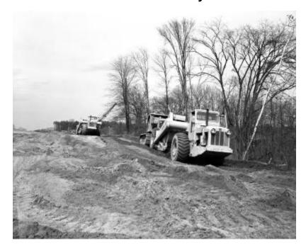
Road grading equipment excavating for the Catskill Thruway in a wooded area of Ulster County. A work truck is also in view. The image is a construction progress photograph taken by the Dept. of Public Works for the Thruway Authority (related photograph file number 5484).
