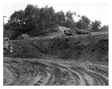
Workmen operating bulldozers and grading equipment, excavating for the Thruway. The image is a construction progress photograph taken by the Dept. of Public Works, Bureau of Construction (related photograph file number 5597).
