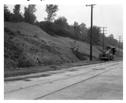
Workman operating a crane, owned by S.A. Scullen, Inc. Construction, moving dirt onto an embankment along a state highway between Mechanicville and Clifton Park (SH 1345). The image is a construction progress photograph taken by the Dept. of Public Works, Bureau of Highways (related photograph file number 5648).
