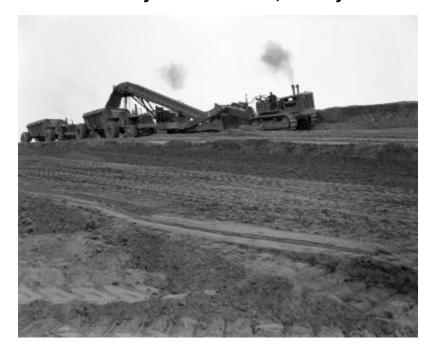
Workmen operating tractors, bottom dump trucks, and other heavy equipment owned by Grandview Construction Corp. of Mt. Vernon, NY, on a site for the NYS Thruway. The image is a construction progress photograph taken for the Dept. of Public Works, Bureau of Highways (related photograph file 5838).
