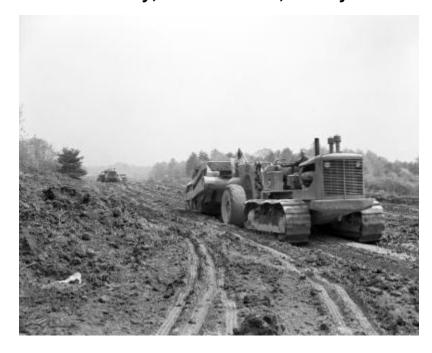
Workman on a crawler tractor pulling a road scraper through a wooded area. Another crawler tractor and scraper, a dump truck, and workmen can be seen in the background. The image is a construction progress photograph taken for the Dept. of Public Works, Bureau of Highways (related photograph file 6028).
