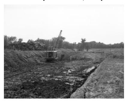
Crane and shovel excavating for the Catskill NYS Thruway Subdivision 5, Albany-Ravena (CT52-8P). The image is a construction progress photograph taken by the Dept. of Public Works, Bureau of Bridge and Grade Crossings. The equipment is owned by Lane Construction Corp., (related photograph file 6108).
