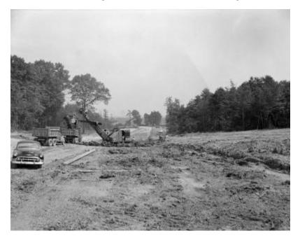
Cable shovel loading dirt into dump trucks for the Catskill NYS Thruway Subdivision 5, Albany-Ravena (CT52-8P). Site is wooded on both sides of the emerging road. Workmen, cars, and a house are also in view. The image is a construction progress photograph taken for the Dept. of Public Works, Bureau of Highways, (related photograph file 6140).
