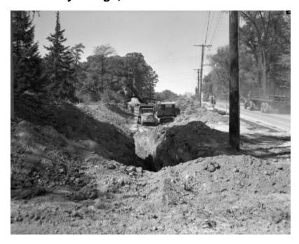
Lorain cable shovel loading dirt into a dump truck alongside state highway 1879. Crewmen, trucks hauling materials, and other heavy equipment are in view. Image is a construction progress photograph taken by the Dept. of Public Works, Bureau of Bridges and Grade Crossings, (related photograph file 6176).
