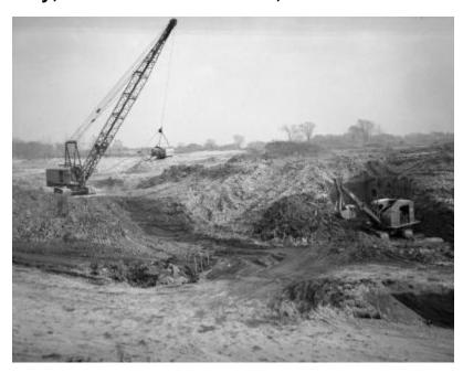
Cable backhoe and crawler crane excavating a site for the New York State Thruway. Image is a construction progress photograph taken by the Dept. of Public Works Bureau of Highways, (related photograph file 6188).
