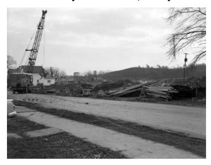
Workmen using a crane to excavate a site for part of the New York State Thruway. Work is being done in a residential area next to houses. The crane is owned by Elmo Hotaling, 4 Orford Street, Albany, N.Y. The image is a construction progress photograph taken by the Dept. of Public Works Bureau of Highways, (related photograph file 6210).
