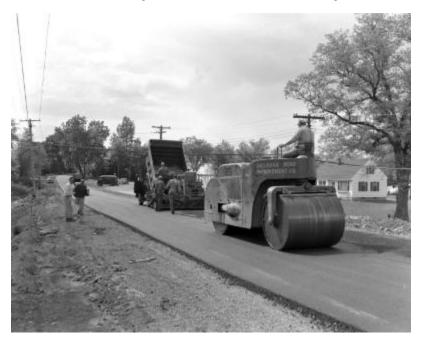
Callanan Road Improvement Company paving part of the Thruway. Crewmen operating a roller and other paving equipment on new asphalt. Houses sit along the roadway. The image is a contruction progress photograph taken by NYS Dept. of Public Works, Bureau of Highways, (related photograph file 6351.)
