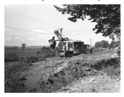
Lorain cable shovel excavating ground at a site for part of the NYS Thruway (project CT528P). The surrounding area is rural. Electrical lines, workmen and a bulldozer are also in view. Image is a construction progress photograph taken by the Dept. of Public Works, Bureau of Highways, (related photograph file no. 6351).
