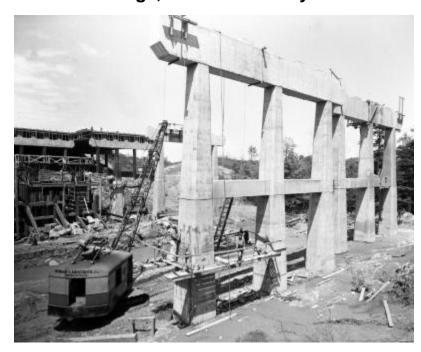
Construction crews erecting a concrete bridge support for the Vloman Kill Bridge on the NYS Thruway. Men can be seen working on scaffolding and operating a crawler crane owned by Munroe-Langstroth, Inc., Norwood, Mass. The image is a construction progress photograph taken by the Dept. of Public Works, Bureau of Highways, (related photograph file 6352).
