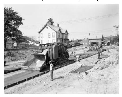
Road crews operating paving equipment, grading, and laying rebar for the NYS Thruway. Several homes and an Esso gas station line the road under construction. The image is a construction progress photograph taken by the Dept. of Public Works, Bureau of Highways, (related photograph file 6383).
