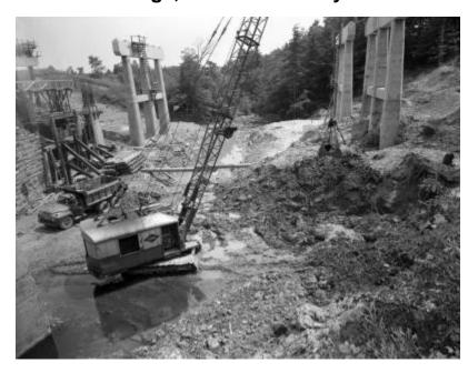
Excavation at the site of the Vloman Kill Bridge on the NYS Thruway. A crawler crane and dump truck can be seen at the base of concrete bridge supports. Land around the site is wooded. The image is a construction progress photograph taken by the Dept. of Public Works, Bureau of Highways, (related photograph file number 6384).
