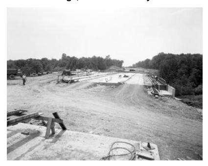
View of the top of the Vloman Kill Bridge under construction on the NYS Thruway. Crewmen and equipment are also in view. The image is a construction progress photograph taken by the Dept. of Public Works, Bureau of Highways, (related photograph file number 6384).
