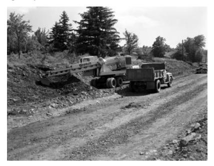
Backhoe, dump truck and car on a road under contruction at Haines Falls in the Town of Hunter. The image is a construction progress photograph taken by the Dept. of Public Works, Bureau of Highways, (related photograph file number 6386).
