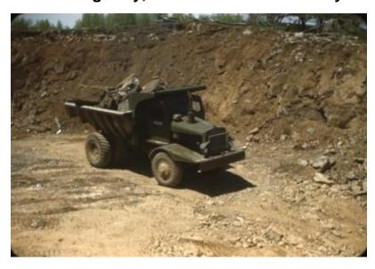
Dump truck full of boulders at an excavated site. Image is a construction progress photograph of NYS Dept. of Public Works project FARC 47-64, state highway 8045, excavating, Broadalbin, East Galway (related photograph file no. 4644).
