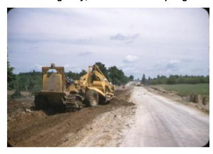
Workman operating a tractor and a motor scraper moving earth for a roadway in Schoharie County. View includes highway under construction, trucks, equipment, crewmen, trees and pastures. Image is a construction progress photograph of Dept. of Public Works project FARC 47-28, State Highway 5569, Sharon-Sharon Springs (related photograph file no. 4670).
