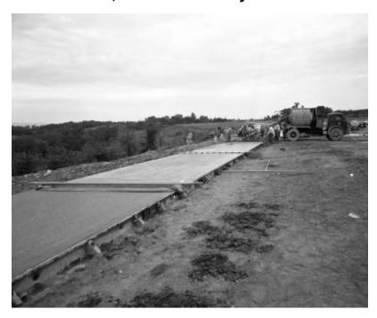
Paving crew pouring and smoothing concrete at a road construction site near Vlomanskill on the NYS Thruway. Cement truck is Ready Mix and Supply Corp., Albany, NY. The image is a construction progress photograph taken by the Dept. of Public Works, Bureau of Highways, (related photograph file number 6469).
