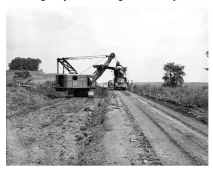
Workmen look on as a cable shovel, owned by Lane Construction Corp., Meriden, Conn., loads a dump truck. The road site is in a rural area, possibly part of NY 32. The image is a construction progress photograph taken for the Dept. of Public Works, Bureau of Highways (related photograph file 6790).
