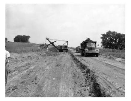
A cable shovel, owned by Lane Construction Corp., Meriden, Conn., scoops earth at a road site in a rural area, possibly NY 32. A dump truck, truck and workmen are also in view. The image is a construction progress photograph taken for the Dept. of Public Works, Bureau of Highways (related photograph file 6790).
