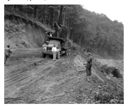
Workmen look on as a cable shovel loads a dump truck, at a state highway site in a wooded area, possibly NY 214. A dump truck and utility trucks are also in view. The image is a construction progress photograph taken for the Dept. of Public Works, Bureau of Highways (related photograph file 6815).
