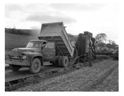
A dump truck, owned by Arute Brothers Contractors, empties crusher onto a road under construction, possibly Route 4. Trucks, paving equipment, workmen, and a hilly landscape are also in view. The image is a construction progress photograph taken for the Dept. of Public Works, Bureau of Highways (related photograph file 6833).
