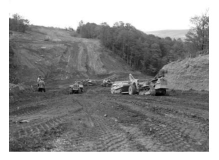
Workmen look on as crawler tractors, bulldozers, and scraper equipment move over a hillside at a road construction site, possibly Route 4. The surrounding landscape is wooded and hilly. The image is a construction progress photograph taken for the Dept. of Public Works, Bureau of Highways (related photograph file 6833).
