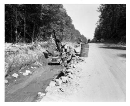
Cable shovels load rock into a dump truck owned by Mayersohn Construction, Albany, NY. Road construction site is in the Adirondacks, possibly Route 28N; pickup trucks are also in view. The image is a construction progress photograph taken for the Dept. of Public Works, Bureau of Highways (related photograph file 6989).
