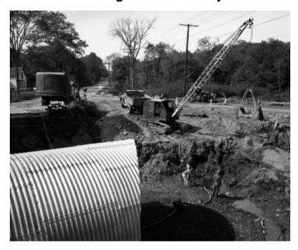
A crawler dragline loads dirt into a dump truck at an excavated site next to a large culvert, possibly for a bridge. Workmen, equipment, a bulldozer, cable shovel, and a house on a rural road are also in view. The image is a construction progress photograph taken for the Dept. of Public Works, Bureau of Bridges (related photograph file 7034).
