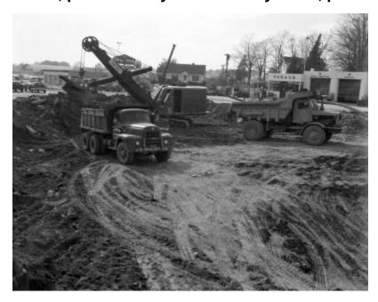
A cable shovel loads dirt into a dump truck owned by J. H. Maloy, Inc., Albany, NY. The construction site may be on Route 9 or 2 in Latham. A Texaco Station, houses, a car lot, shopping mall, several utility trucks and another dump truck can also be seen. The image is a construction progress photograph taken for the Dept. of Public Works, Bureau of Highways (related photograph file 7052).
