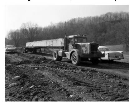
Truck and flatbed trailer transporting building material for a bridge at a location in Herkimer County described as Uebler Road. The truck is on a dirt road; two cars are also in view. The image is a construction progress photograph taken for the Dept. of Public Works, Bureau of Bridges (related photograph file 7071).
