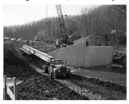
Truck and flatbed trailer transporting material for a bridge under construction at a site described as Uebler Road. The truck is on a dirt road beside a new bridge abutment. A crane, workmen, trucks, cars, dump truck, tractor, and second truck and flatbed trailer transporting material are also in view. The image is a construction progress photograph taken for the Dept. of Public Works, Bureau of Bridges (related photograph file 7071).
