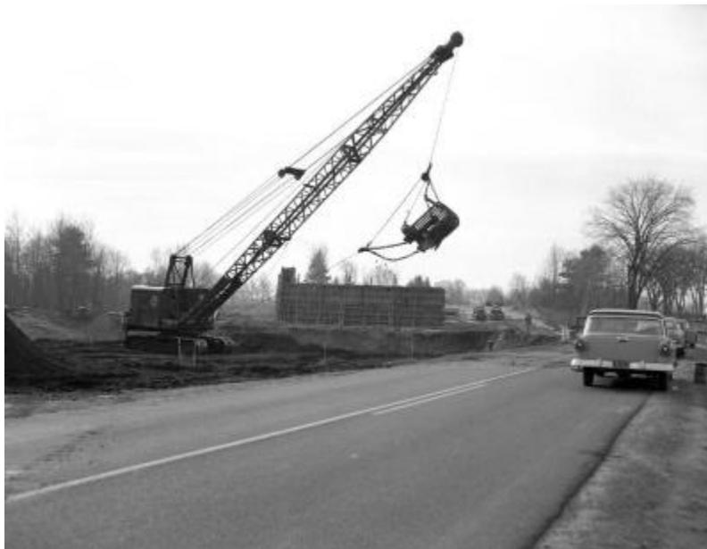
Crawler dragline at a construction site in Saratoga. The excavated site is next to a paved highway; a workman, cars, trucks, equipment, and woods are also in view. The image is a construction progress photograph taken for the Dept. of Public Works, Bureau of Bridges (related photograph file 7099).
