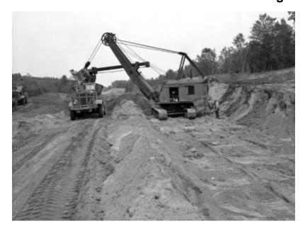
Cable shovel loading dirt into a dump truck at an excavation site in a wooded area of Saratoga County; another dump truck and workmen are also in view. The image is a construction progress photograph taken for the Dept. of Public Works, Bureau of Bridges and Railroad Grade Crossings (related photograph file 7220).
