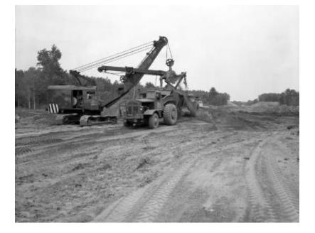
Cable shovel loading dirt into dump trucks at an excavation site in a wooded area of Saratoga County. The image is a construction progress photograph taken for the Dept. of Public Works, Bureau of Bridges and Railroad Grade Crossings (related photograph file 7220).
