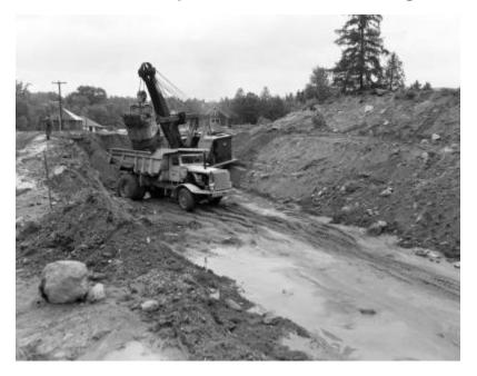
Bucyrus-Erie cable shovel loading earth into a dump truck at a road construction site in the Adirondacks, possibly Route 28N. Forest and several houses are also in view. The image is a construction progress photograph taken for the Dept. of Public Works, Bureau of Highways (related photograph file 7447).
