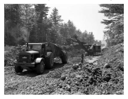
Workmen operating a cable shovel and bottom dump truck at a road construction site in the Adirondacks, possibly Route 28N. The image is a construction progress photograph taken for the Dept. of Public Works, Bureau of Highways (related photograph file 7742).
