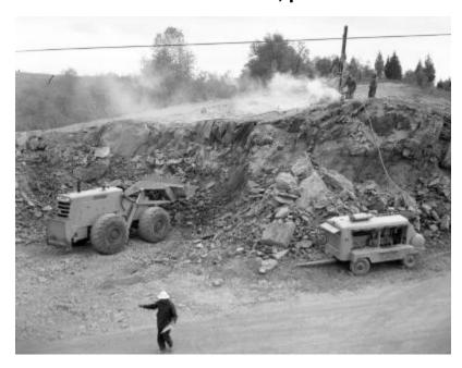
Two workmen operate a generator and drill to break up a rocky embankment while another uses a shovel loader to move debris; a fourth directs from below. The image is a construction progress photograph taken by the Dept. of Public Works, Bureau of Highways (related photograph file number 7983).
