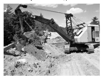
Detail of a P&H cable shovel in operation at a road construction site (possibly NY Route 86) in the Adirondacks. The image is a construction progress photograph taken by the Dept. of Public Works, Bureau of Highways (related photograph file number 8046).
