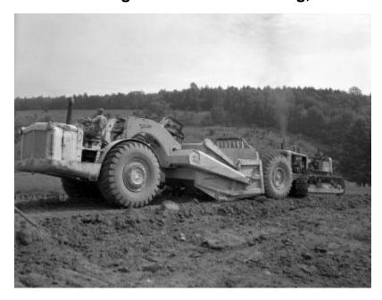
Workmen operating a Euclid motor scraper and bulldozer at a road construction site (possibly Route 9N) in the Adirondacks. The project includes Ticonderoga Village, part 2; Ticonderoga to Crown Point; and Schroon Lake to Ticonderoga. The image is a construction progress photograph taken by the Dept. of Public Works, Bureau of Highways (related photograph file number 8074).
