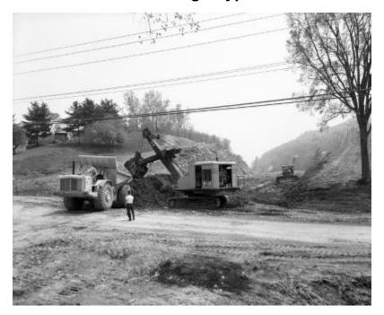
A workman looks on as a cable shovel loads a dump truck with earth excavated from the construction site for the Ticonderoga Bypass or the NY 9N and NY 22 overlap. A bulldozer is also in view. The excavated site is in a wooded area. The image is a construction progress photograph taken by the Dept. of Public Works, Bureau of Highways (related photograph file number 8246).
