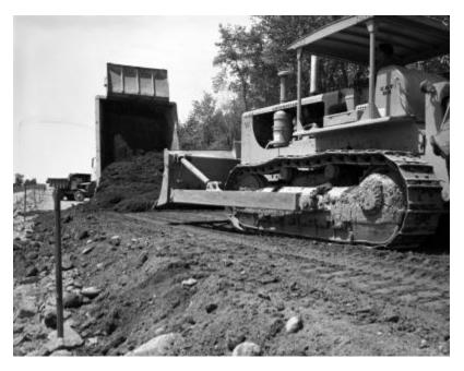
Bulldozer spreading earth unloaded by a dump truck during construction of highway no. 817 Scotch Church - Blue Corners, in the town of Charlton. The image is a construction progress photograph taken by the Dept. of Public Works, Bureau of Highways (related photograph file number 8263).
