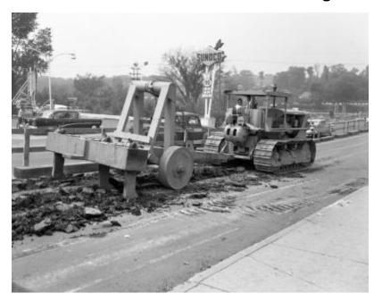
Workman using a crawler machine to pull road removal equipment over a roadway in a residential area of Glens Falls. A Sunoco gas station, customers, cars, a house, and a multi-story building are in the background. The image is a construction progress photograph taken by the Dept. of Public Works, Bureau of Highways (related photograph file number 8329).
