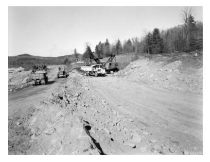
View of an area in the Adirondacks under excavation for a new road. Men work on the ground and operate a cable shovel (Lane Construction Corp., Meriden, Conn.), dump trucks, and shovel trucks. Forest and mountains surround the area. The image is a construction progress photo taken by the NYS Dept. of Public Works, Bureau of Highways (related photograph file 9092).
