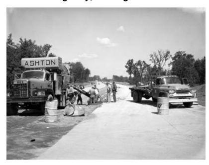
Crew pouring ready mix onto a highway under construction in Saratoga County. A ready mix truck (owned by Ashton), a utility truck and eight crewmen are in the foreground; stretch of tree-lined highway, equipment, cars and trucks in the background. The image is a construction progress photograph taken by the Dept. of Public Works, Bureau of Highways (related photograph file number 9413).
