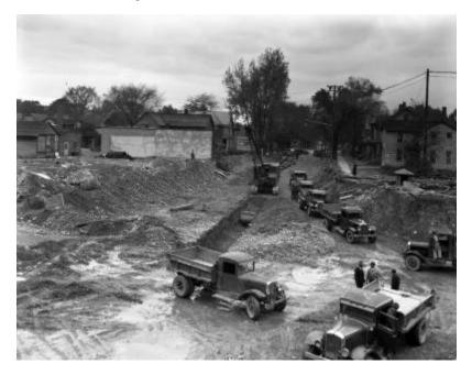
Railroad construction, possibly on South Main Street in Elmira. A crawler crane is digging up the street and several workmen and trucks are on site. A sign for Keefe Grocery Co. is on one of the buildings along the residential tree-lined street in the background. The project is associated with Public Service Commission number 3200. The image is a construction progress photograph taken by the Dept. of Public Works (related photograph file number 1031).
